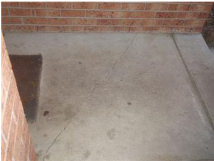
Porch Concrete Movement noted in concrete infill slab Concrete is not connected or is part of the dwellings foundations No concern
