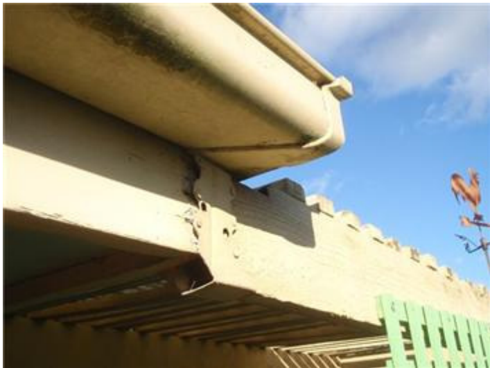
Porch Concrete Movement noted in concrete infill slab Concrete is not connected or is part of the dwellings foundations No concern
