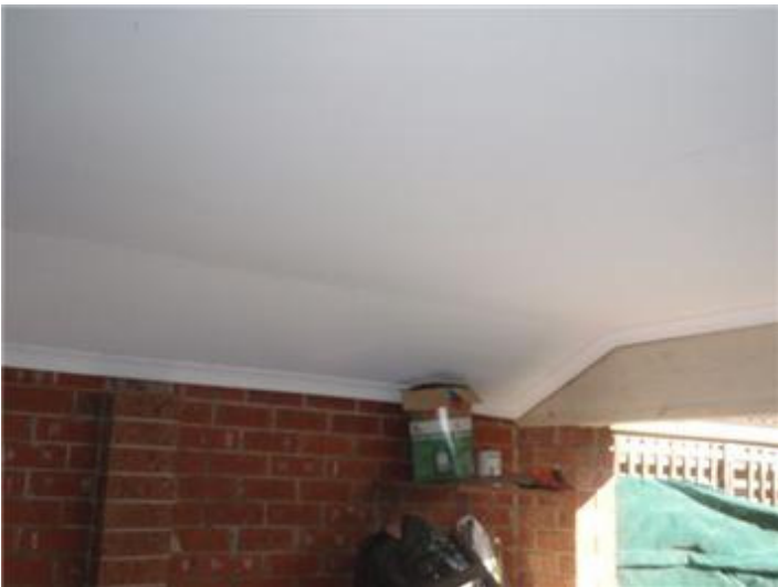
Garage Ceilings Plaster Minor movement noted between plaster sheets at join, minor repairs required and is unknown if they will return Ceiling has come away from ceiling joists in areas and may require re fixing in the near future Cost $300
