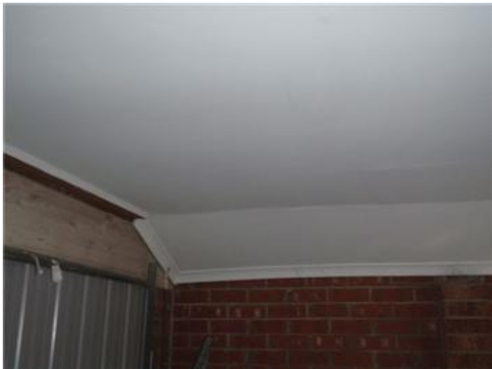
Garage Ceilings Plaster Minor movement noted between plaster sheets at join, minor repairs required and is unknown if they will return Ceiling has come away from ceiling joists in areas and may require re fixing in the near future Cost $300
